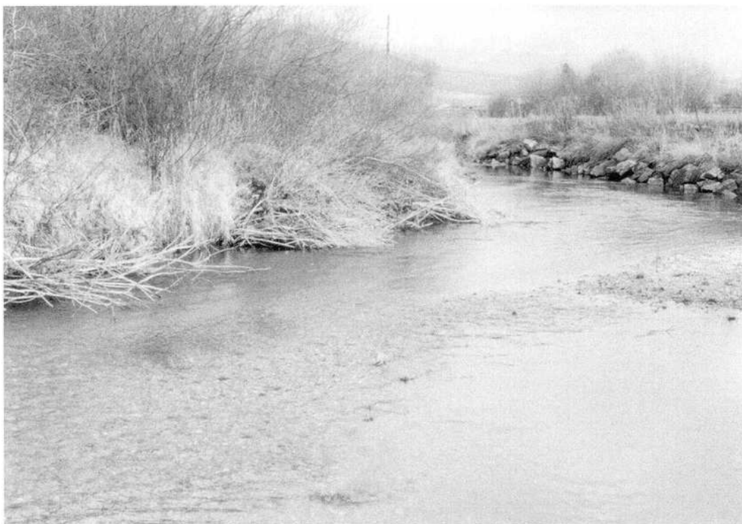
Figure 2. In this undisturbed streambank in the foreground and a riprapped streambank in the background, note the absence of low overhead cover, undercut bank and potential for woody debris recruitment of the riprapped bank compared to the undisturbed bank.
