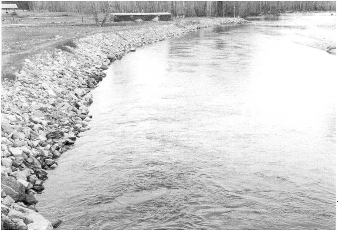
Figure 1. This conventional riprap project is on the Bitterroot River, Montana.
