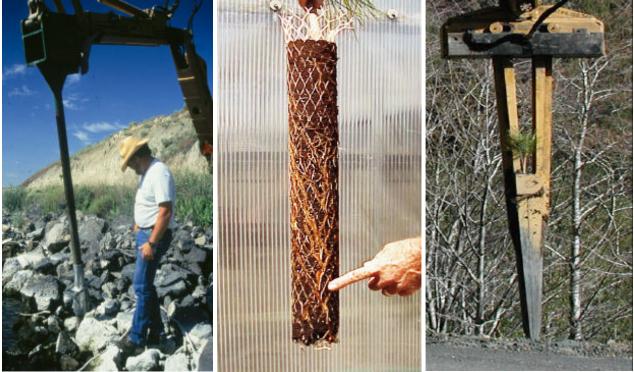
Figure 7. Conventional stinger application (left) and new stinger design (right) that uses soil-encapsulated plants (center) for insertion into riprap sections
