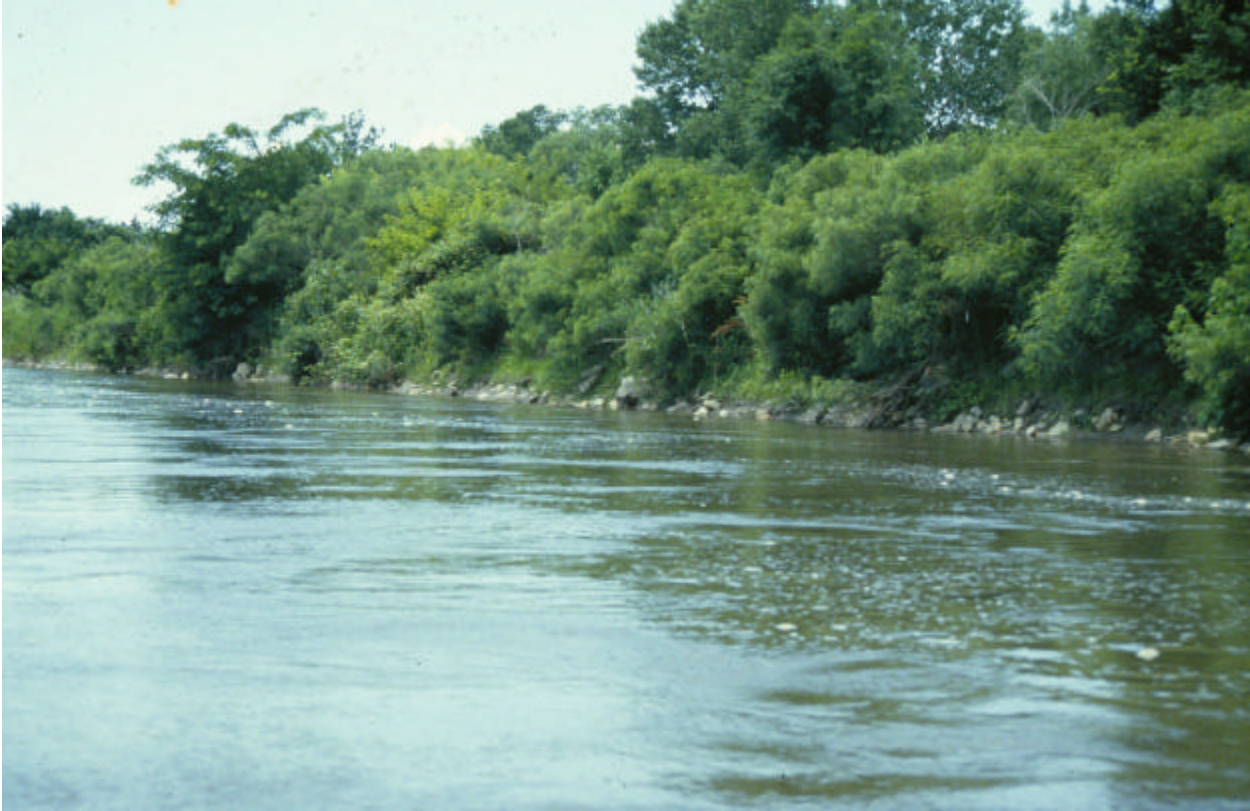
Figure 6. A combination of riprap in the toe section and woody vegetation on the upper banks often affords the best combination of stabilization and environmental benefits
