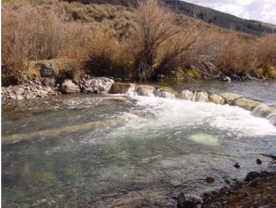
Figure 8. Low-head stone weir on the North Fork of the White River, Colorado
