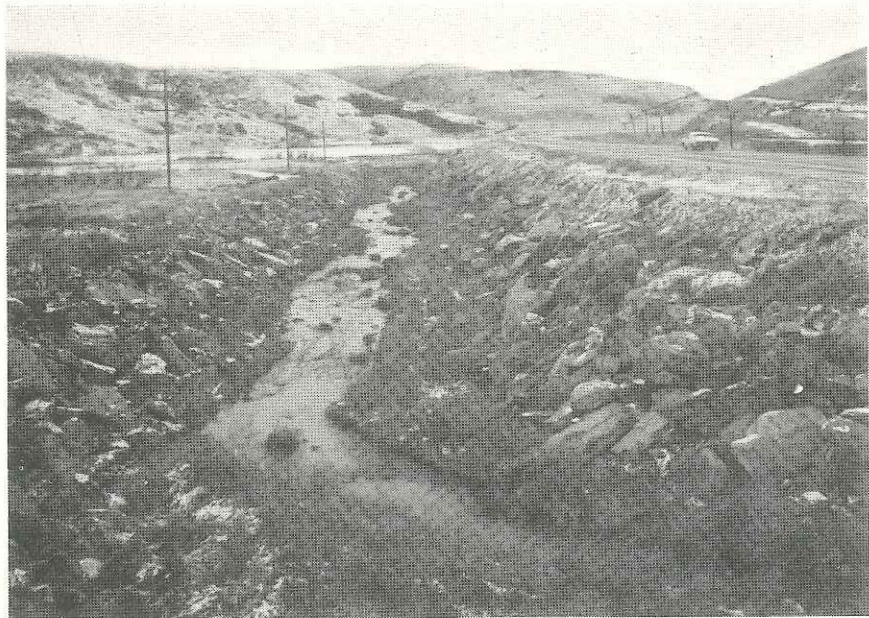
A CHANNEL RELOCATION ON OTTER CREEK NEAR BELT. Nearly one-fourth of this stream had been altered.
